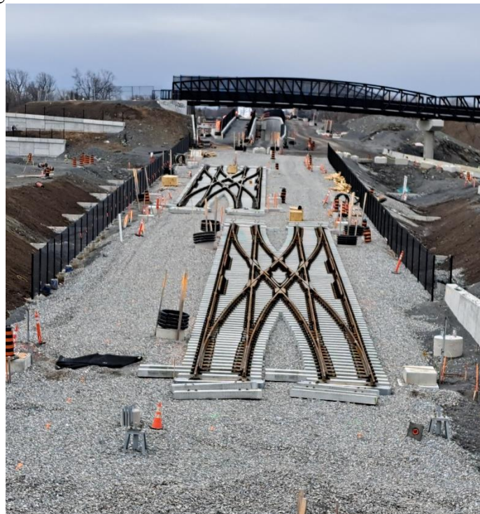
Figure 1: Turnouts and diamond crossings under construction
